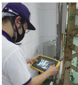
Air leak investigation
