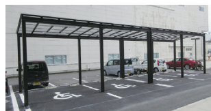
Parking for wheelchair users (West Main Building, Gunma Plant)
