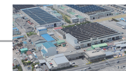
Utsunomiya South Plant/2nd South Plant
